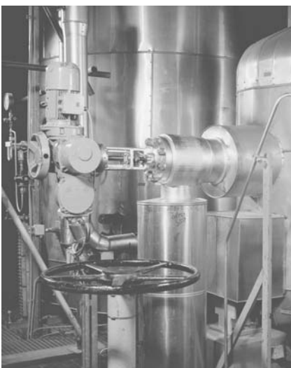
H.P. preheater in a nuclear power station equipped with a condensate drain control valve type ZK 29
